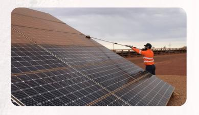
The build-up of dust on panels can have a notable impact on efficiency and dependability, potentially resulting in communication system malfunctions and decreased mine production output.
